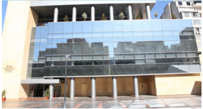
Wassef and Souad Sawwaf Building and Extension
